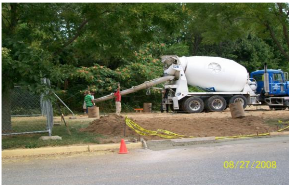
The cement truck arrived on the second day of construction.
