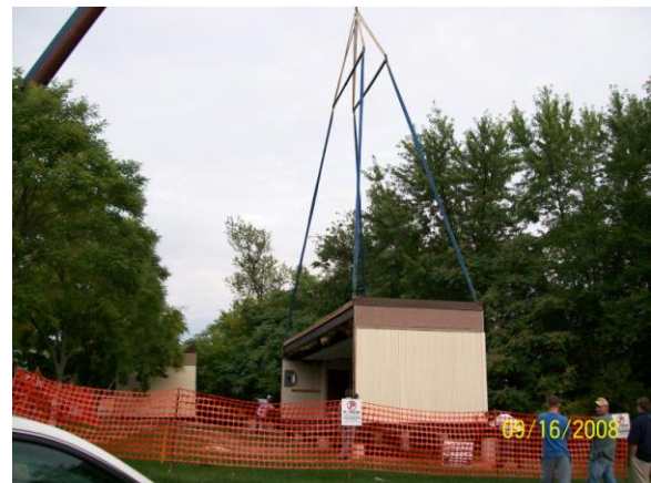
The back half is being lowered onto the foundation.
